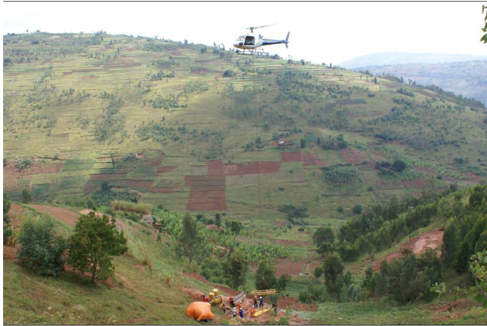
Figure 10.1.1_1 Disassembled Drill Rig Being Moved to Site by Helicopter
